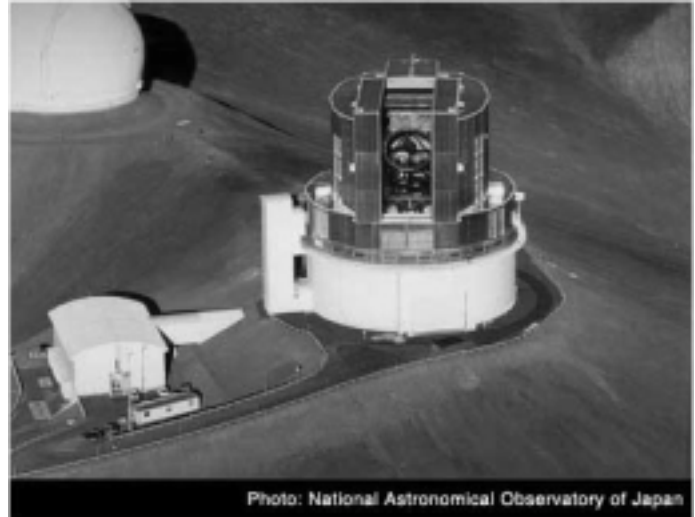
Fig. 1. Enclosure of the 8.2m Subaru Telescope at the summit of Mauna Kea, Hawaii.
